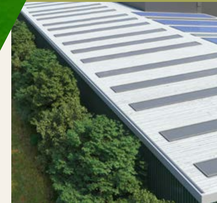
Landscaping & PV provision at SEGRO Park Tottenham
