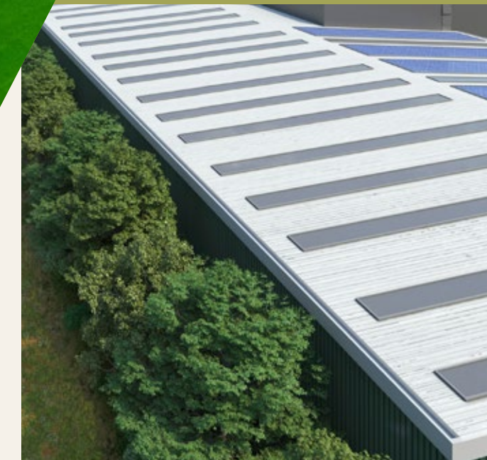
Landscaping & PV provision at SEGRO Park Tottenham
