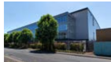
Data Centre, Slough Trading Estate, UK
