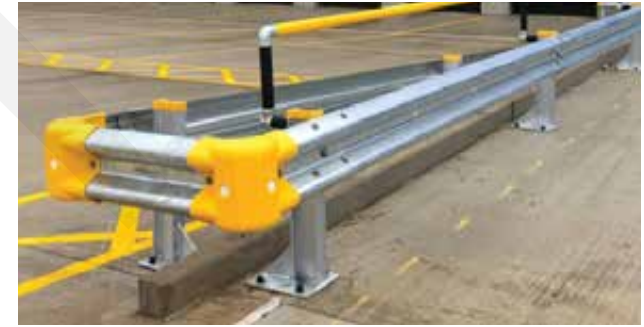
Service Yard - Barrier protection & Safety lining
