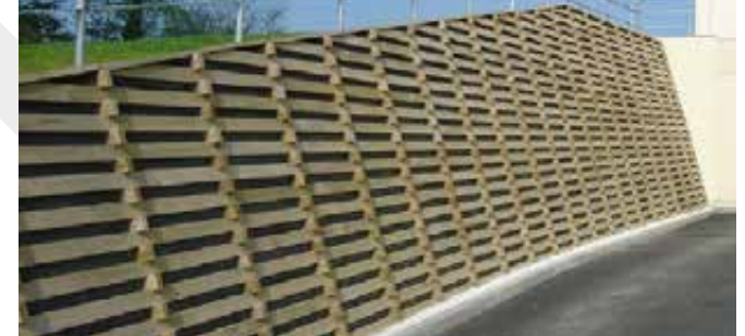
Cribblock retaining wall
