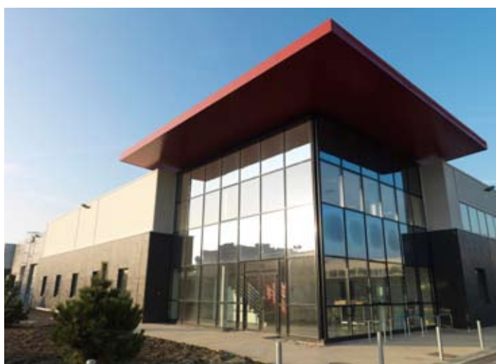
Following the success of rainwater harvesting schemes at La Courneuve (pictured), Gonesse and Marly La Ville, we are incorporating a similar scheme for our new logistics building at Gonesse.
