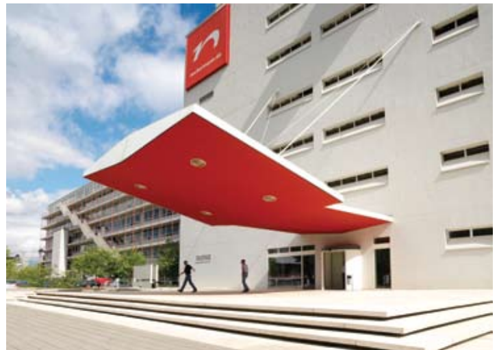
At our Neckermann site in Frankfurt, 7,000 sq m of photovoltaic panels installed through an agreement with Juwi Solar generated 150,000 kWh, providing us with rental income and our occupier Neckermann with access to clean power at preferential rates.
