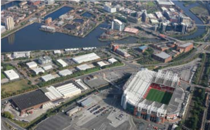
At Trafford Park in Manchester, we are working with occupier AKW Group to reduce carbon emissions by improving insulation on 5,500 sq m of roof space, as well as installing automatic motion sensors on lighting.
