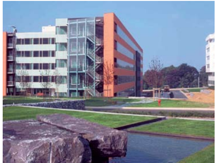
At Pegasus Park in Brussels, we are replacing traditional lighting with energy-efficient LED alternatives.
