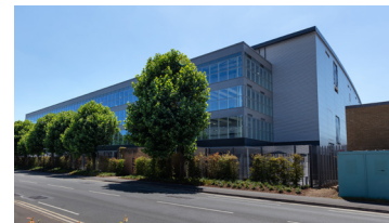
Data Centre, Slough Trading Estate, UK
