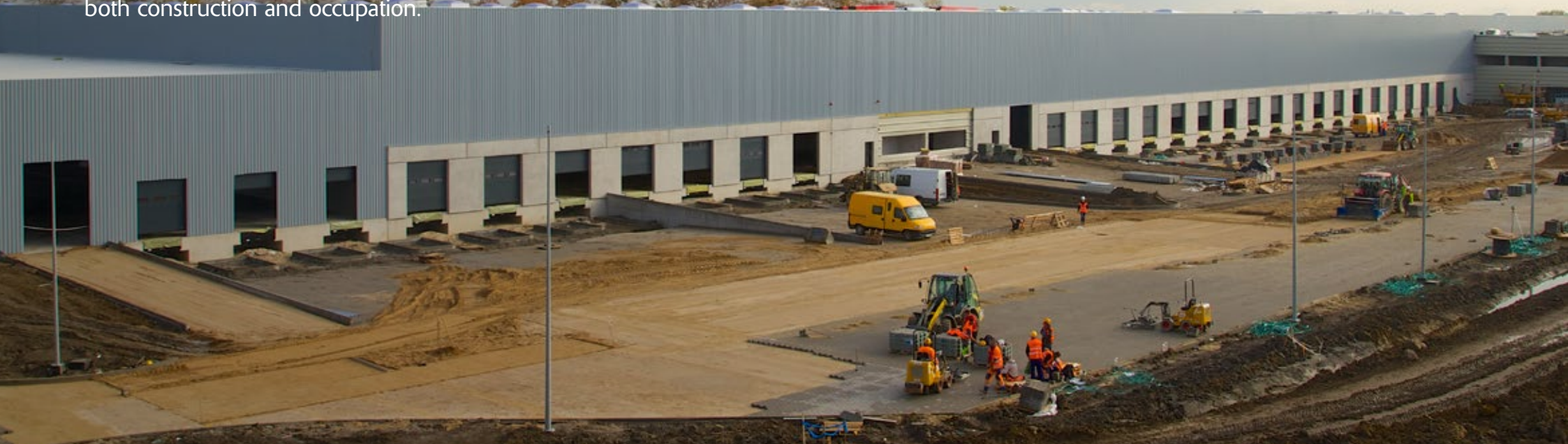
IMAGE: CONSTRUCTION AT SEGRO LOGISTICS PARK GDANSK / POLAND
